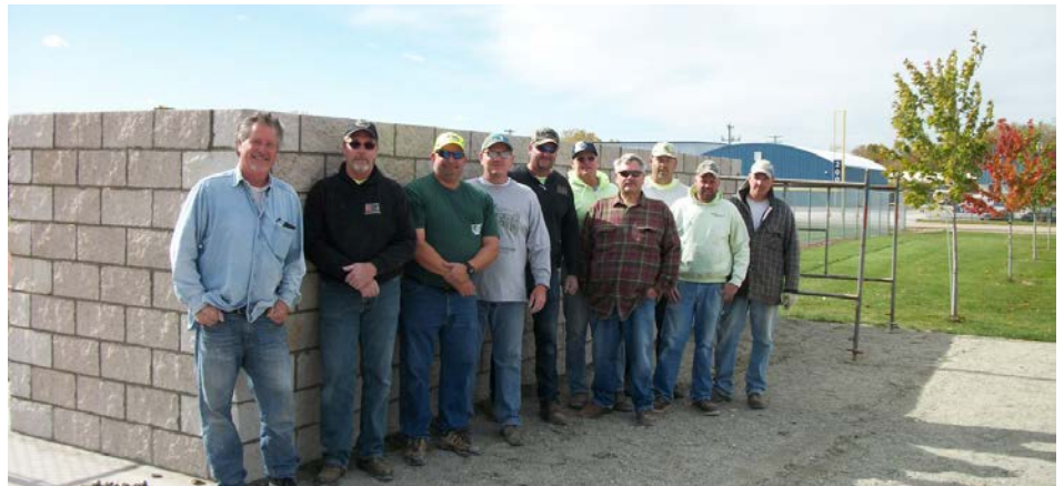
Bricklayers and Allied Craftworkers (BAC) and Laborers' Local 330 giving back to the community by building two dugouts for Menasha youth sports. Miron Construction donated the equipment.
